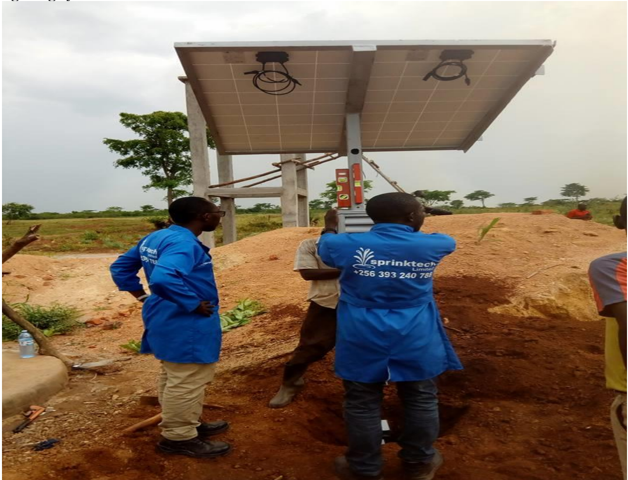
Our team installing a solar water pumping system
