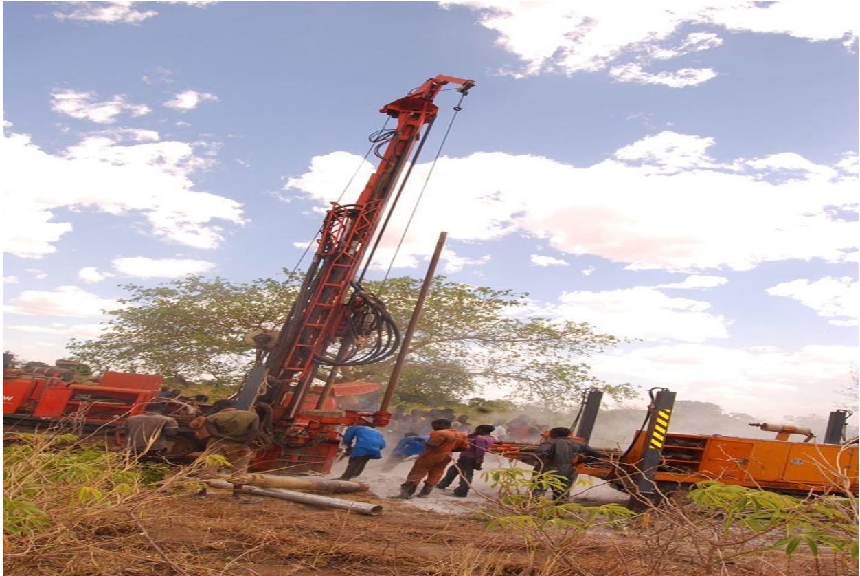
Our drilling rig in action
